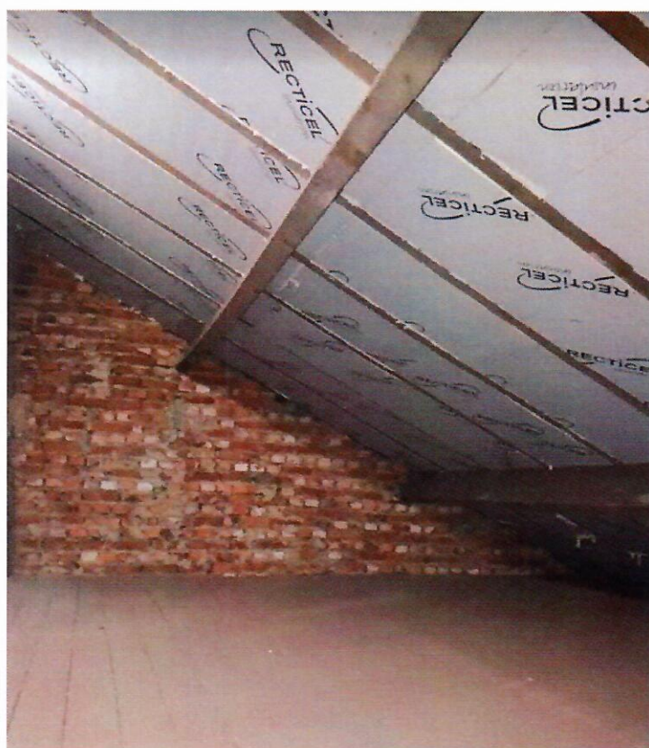
Dak woning: Eurowall PUR 600x1200x60mm + dampscherm folie + 18mm OSB
